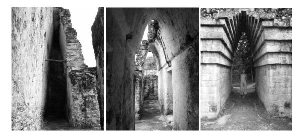
Figure 3.6. Examples of the Maya vault system. As seen, they vary slightly in shape but remain constant in their basic construction, which consists of two sloping walls rising until they meet at the peak. Photographs taken by author.
