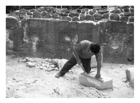
Figure 3.1. Worker at the site of Tikal, Guatemala, trimming blocks for use in restoration of architecture. Photograph taken by author.
