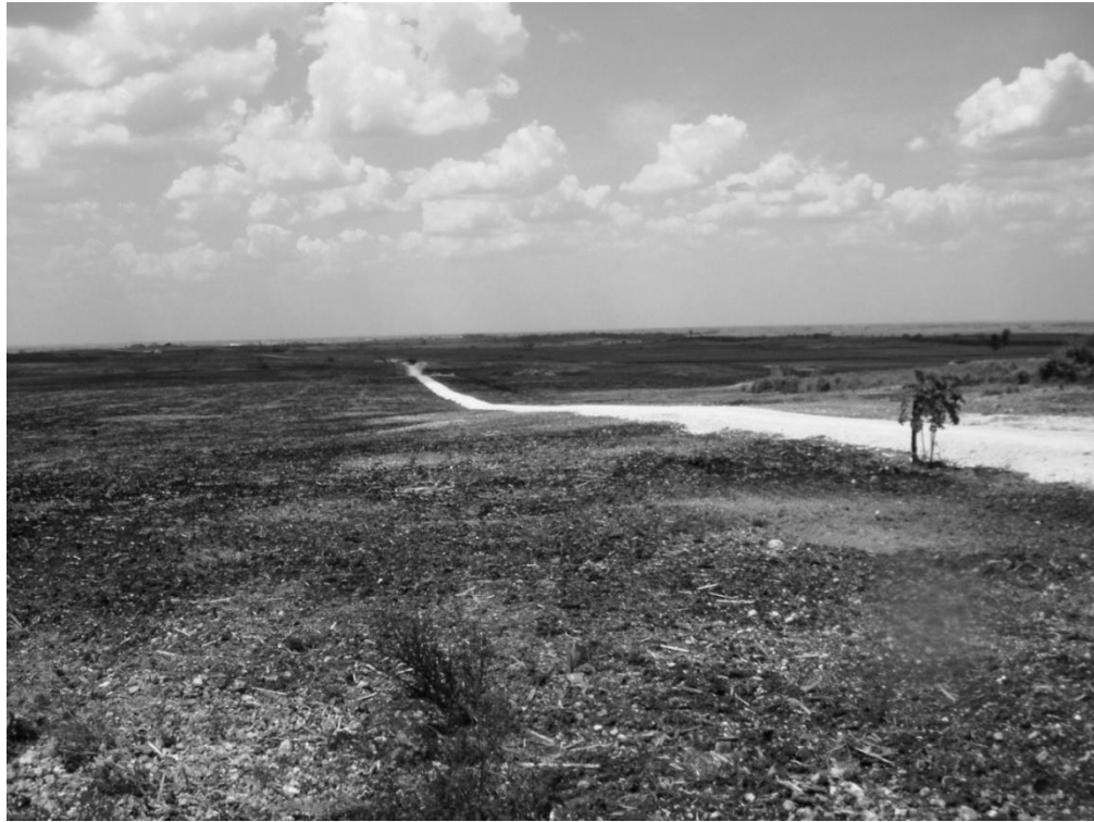
Figure 72: Construction of a Road in the Settlement Zone
