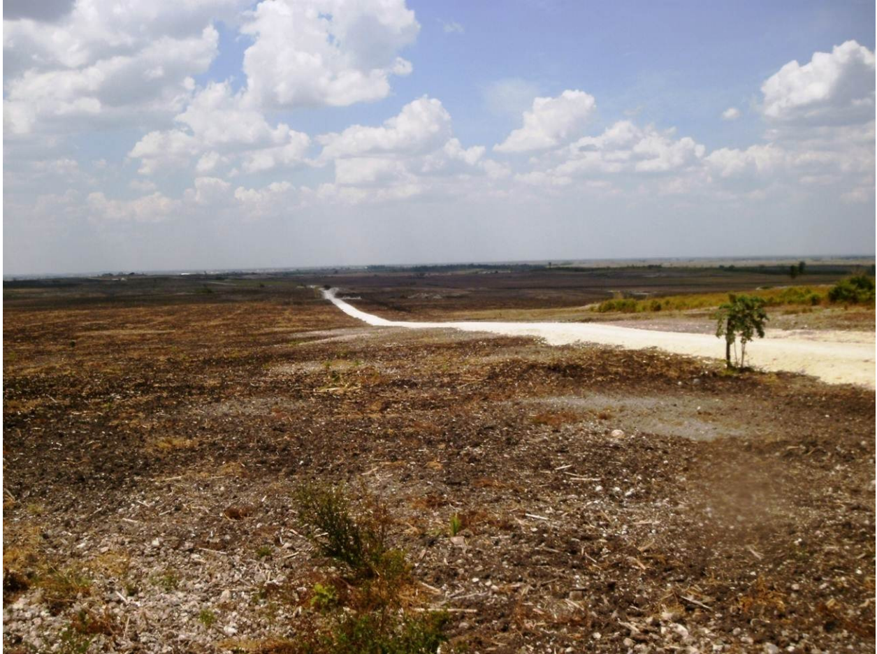
Figure 4-3: Construction of a Road in the Settlement Zone
